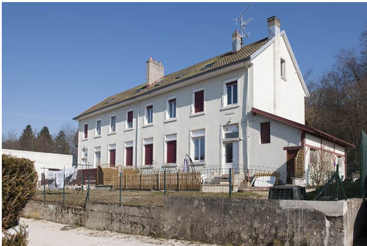
Ecole. Façade ouest.
