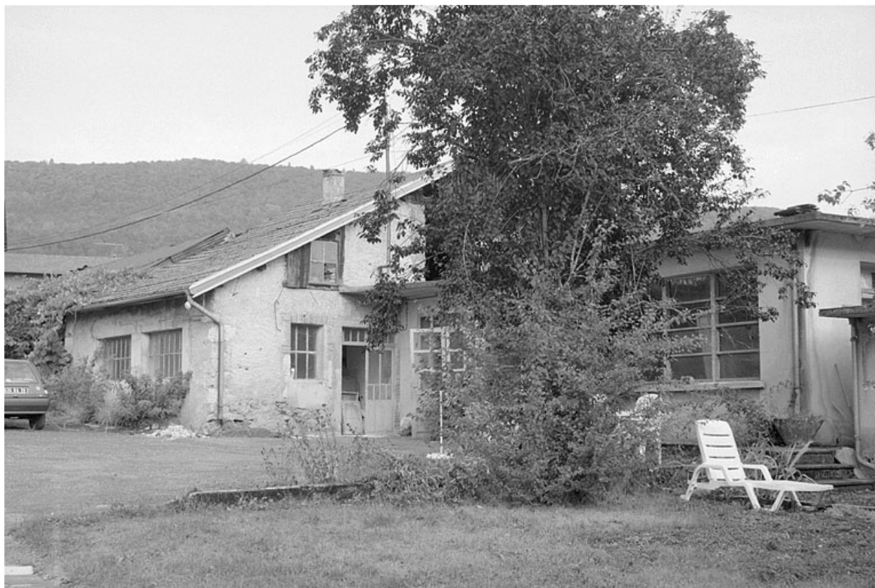
Ateliers de fabrication (E, F).
