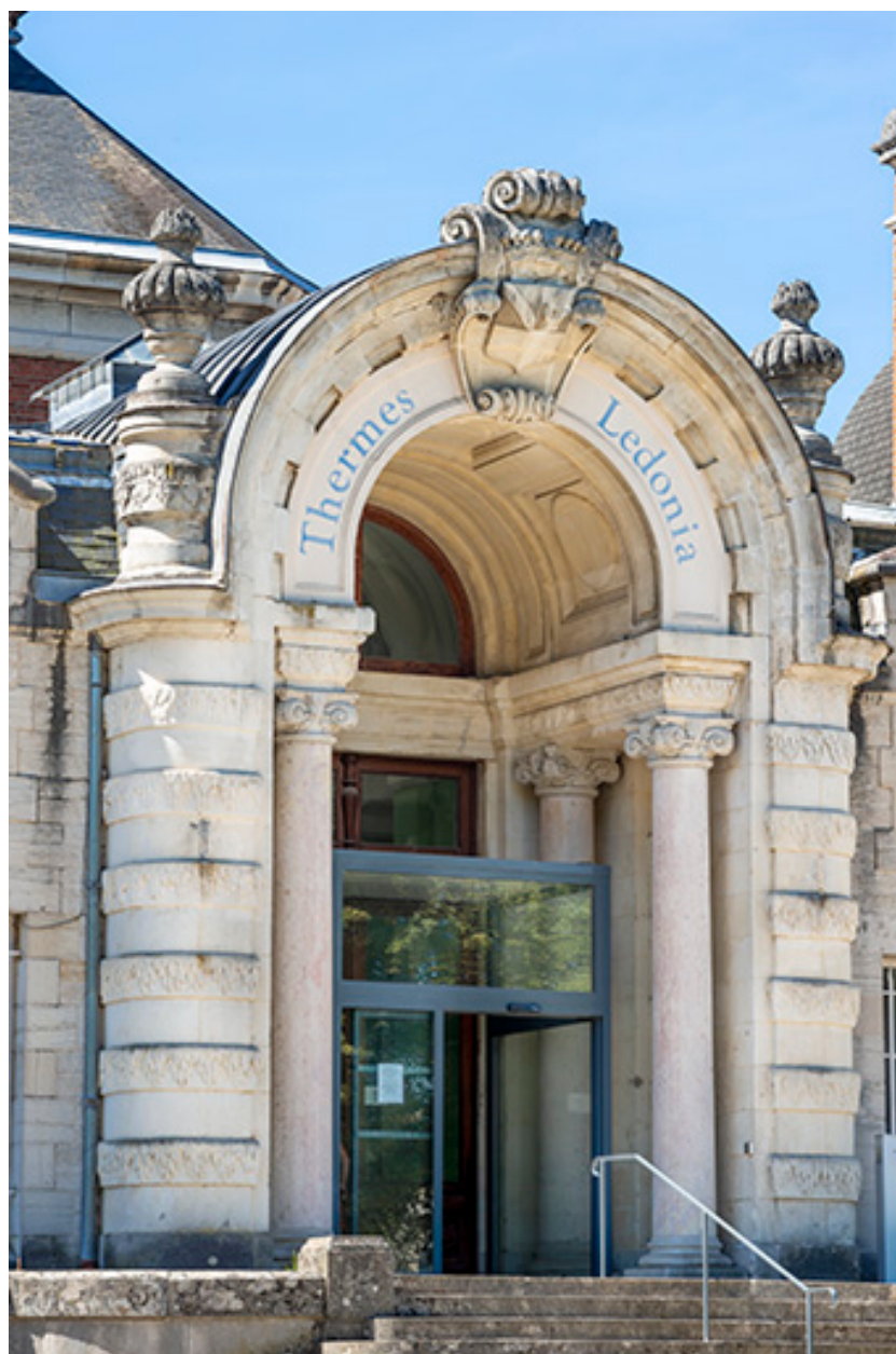
Façade principale, portail.
