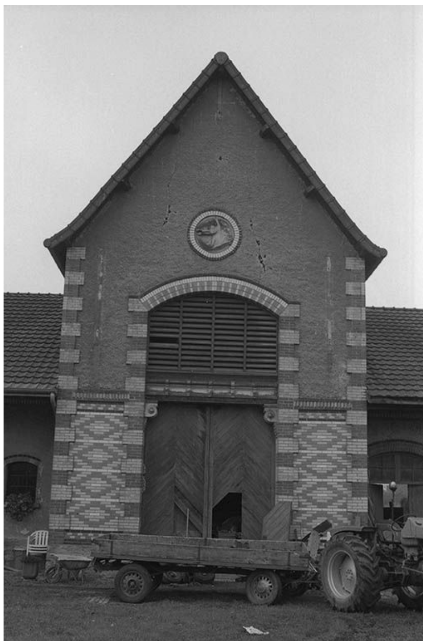
Corps central, façade est.
