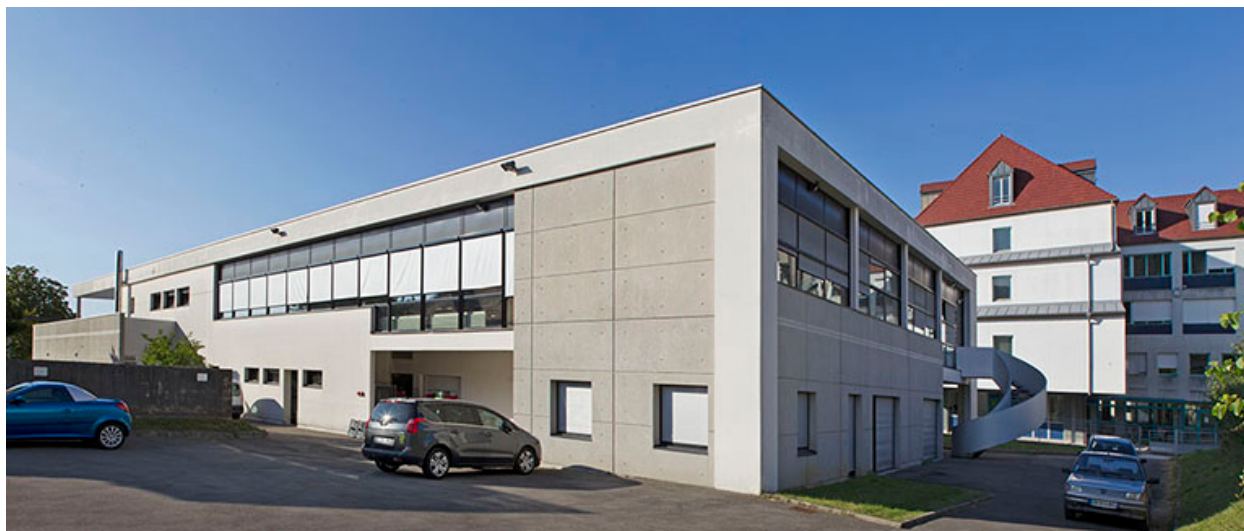
Restauration : façade Est.
