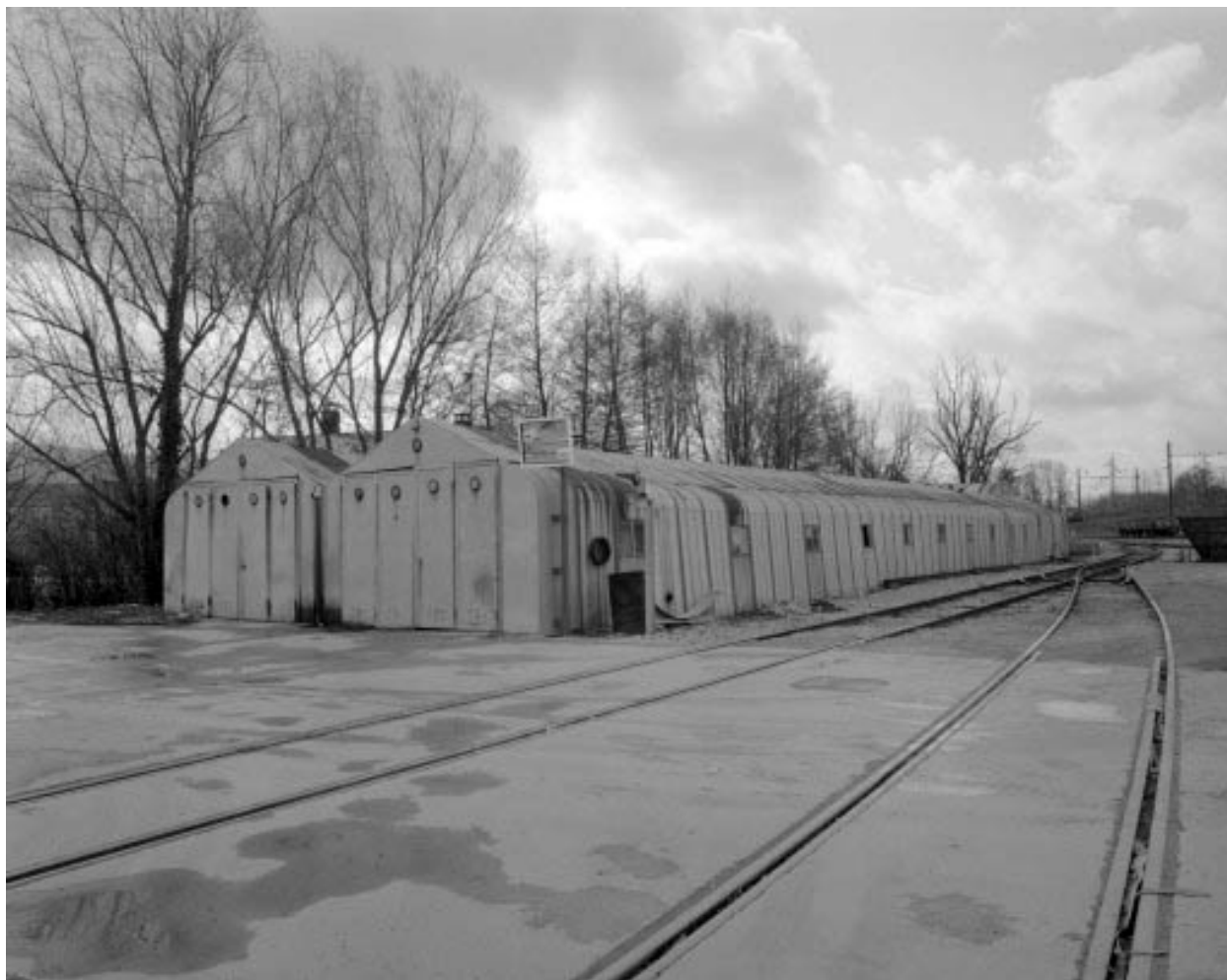
Baraques de chantier (F).
