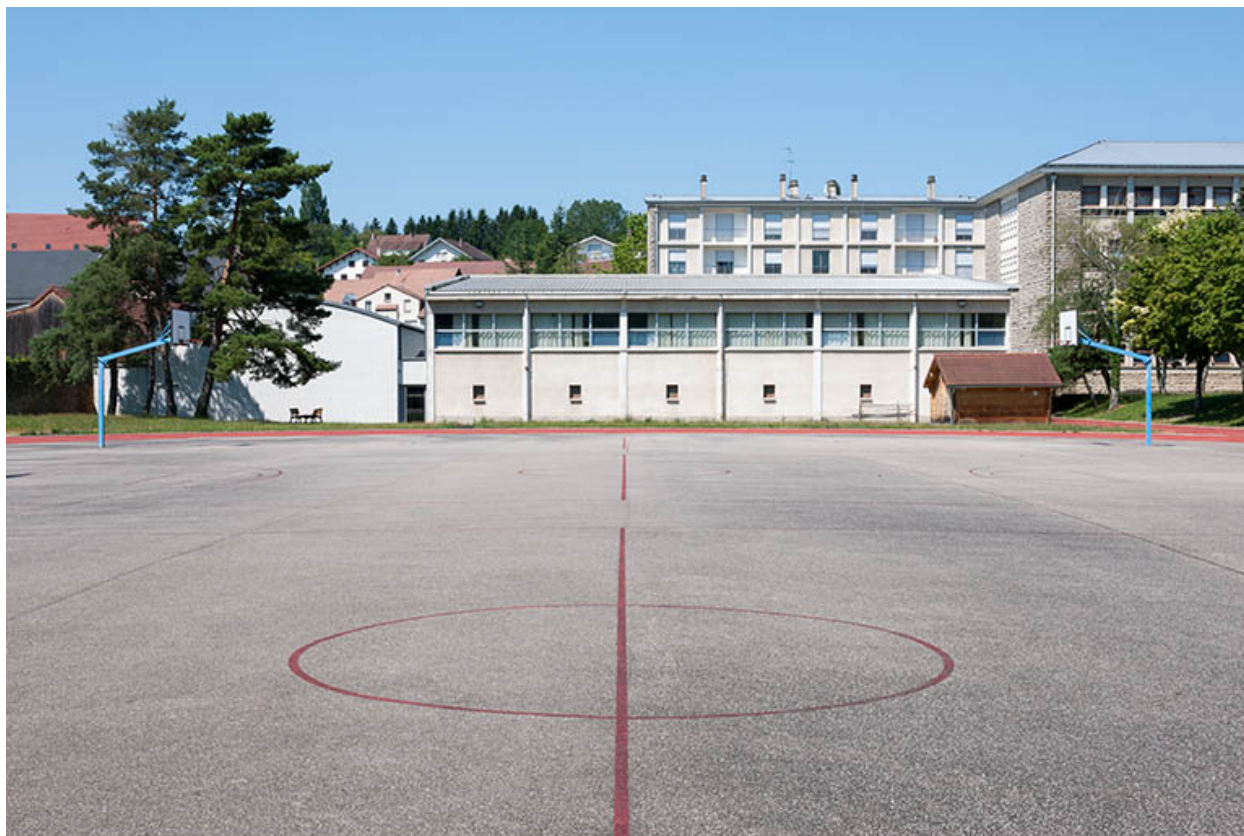
Gymnase et installations sportives.
