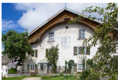
Façade antérieure. Phot. Sonia Dourlot IVR43_20152500791NUC2A
