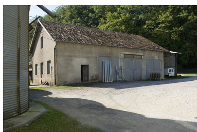
Garage. Phot. Jérôme Mongreville IVR43_20067000875NUCA
