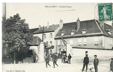
Arc-lès-Gray. - Fonderie Dagot. Phot. Jérôme Mongreville IVR43_20097000071NUC2A
