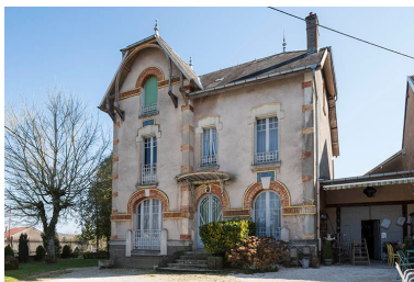
Façade principale. Phot. Jérôme Mongreville IVR43_20177000206NUC4A
