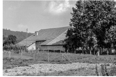
Façade postérieure. Phot. Gilbert Poinot IVR43_19752501248Z
