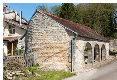
Mur pignon du lavoir. Phot. Sonia Dourlot IVR43_20167000527NUC4A
