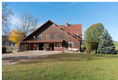
Façade antérieure (sud). Phot. Sonia Dourlot IVR43_20172501656NUC4A
