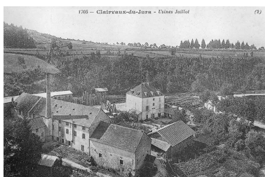
Clairvaux-du-Jura - Usines Jaillot. Phot. Jérôme Mongreville IVR43_19963900003X
