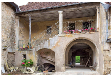
Façade postérieure. Phot. Sonia Dourlot IVR43_20157000328NUC2A
