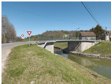
Le pont. Phot. Thierry Kuntz IVR26_20122102747NUC4A
