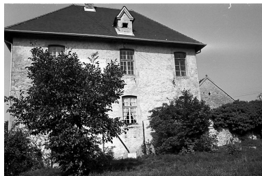
Façade postérieure. Phot. Gilbert Poinot IVR43_19762500908Z
