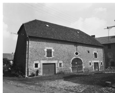
Parties agricoles en 1980. Phot. Dominique Dominguez IVR43_19803900285X
