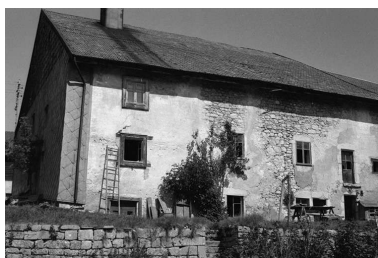
Façade postérieure. Phot. Gilbert Poinot IVR43_19752501021Z
