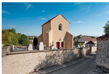
Façade. Phot. Pierre-Marie Barbe-Richaud IVR26_20122101467NUC4AQ
