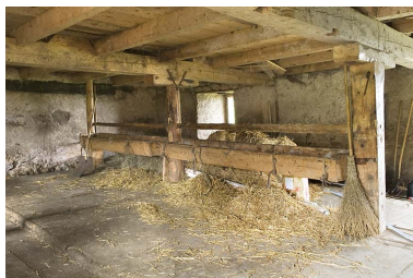
Etable. Phot. Jérôme Mongreville IVR43_20082500939NUC2A
