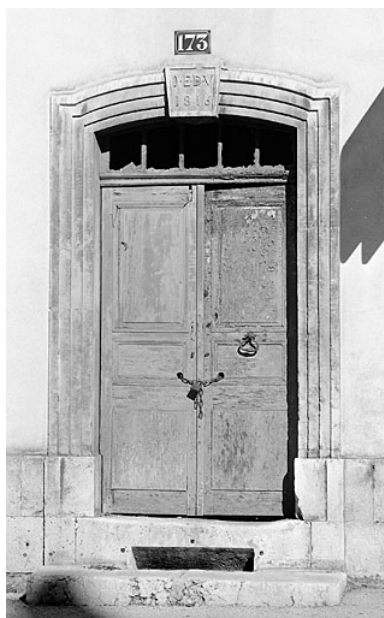
Entrée principale. Phot. Yves Sancey IVR43_20033900496X
