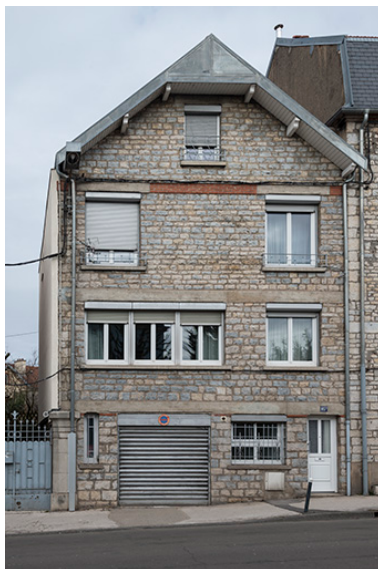
Mur-pignon sud. Phot. Jérôme Mongreville IVR43_20182500527NUC4A
