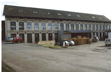
Atelier de fabrication est. Phot. Yves Sancey IVR43_20009000711ZA
