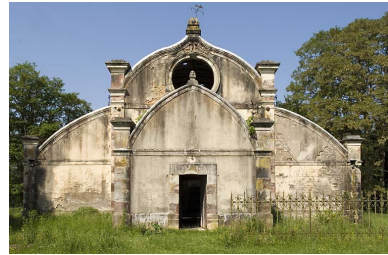
Serre. Mur-pignon est. Phot. Jérôme Mongreville IVR43_20077000300NUCA
