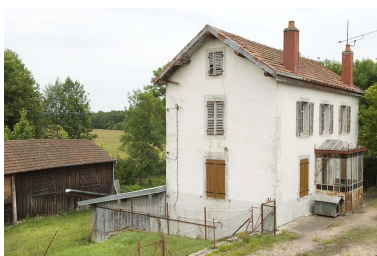
Logement patronal. Phot. Jérôme Mongreville IVR43_20097000368NUC2A
