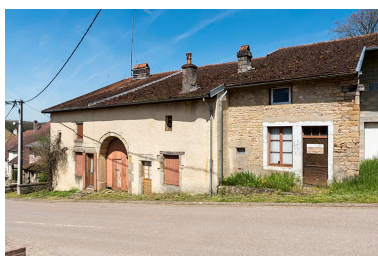
Fermes, Grande rue. Phot. Sonia Dourlot IVR43_20167000565NUC4A
