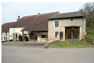
Fermes, Grande rue. Phot. Sonia Dourlot IVR43_20167000546NUC4A
