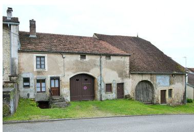
fermes , Grande rue. Phot. Sonia Dourlot IVR43_20167000635NUC4A
