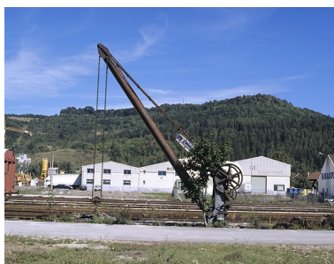
Grue. Phot. Yves Sancey IVR43_20043900155XA
