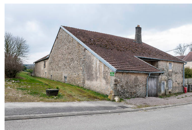
Mur pignon. Phot. Jérôme Mongreville IVR43_20167000239NUC4A
