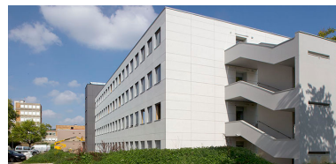
Internat : façade sud. Phot. Sonia Dourlot IVR43_20143900674NUC2A
