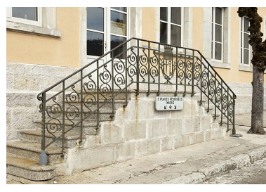
Perron. Phot. Jérôme Mongreville IVR43_20092501642NUC2A
