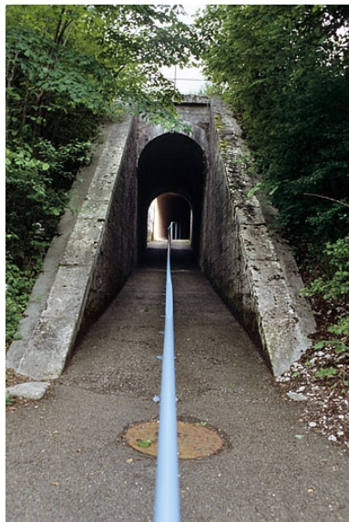
Tête aval (nord). Phot. Yves Sancey IVR43_20053900859ZA
