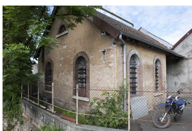
Chaufferie (?). Phot. Jérôme Mongreville IVR43_20122500962NUC4A
