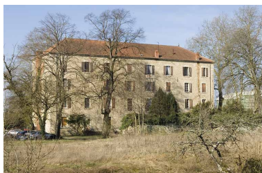
Façade est. Phot. Jérôme Mongreville IVR43_20097000198NUC2A
