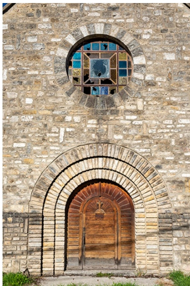
Baies du mur-pignon est. Phot. Jérôme Mongreville IVR43_20223900869NUC4A
