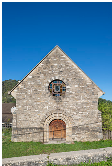
Mur-pignon est. Phot. Jérôme Mongreville IVR43_20223900866NUC4A
