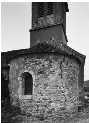
Abside. Phot. Michel Thierry IVR26_19782100860V
