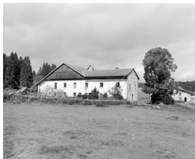
Facade antérieure. Phot. Yves Sancey IVR43_19772500358X
