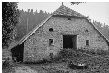
Façade postérieure. Phot. Gilbert Poinot IVR43_19752501324Z
