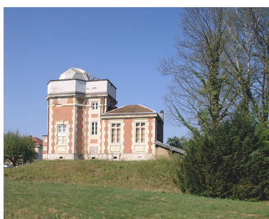
Façade est. Phot. Jérôme Mongreville IVR43_20022501155XA
