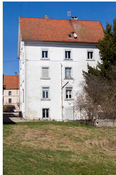
Façade postérieure. Phot. Sonia Dourlot IVR43_20152500880NUC2A
