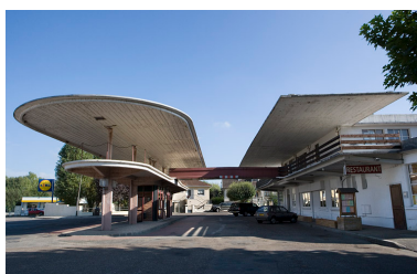
Gare et station bus. Phot. Yves Sancey IVR43_20067000891NUCA
