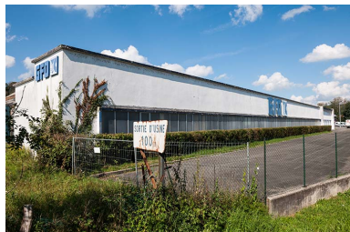
Façade est. Phot. Jérôme Mongreville IVR43_20142501382NUC4A
