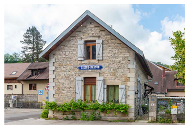
Façade est. Phot. Jérôme Mongreville IVR43_20243900703NUC4A
