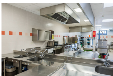
Cuisine d'application. Phot. Jérôme Mongreville IVR43_20143900432NUC4A
