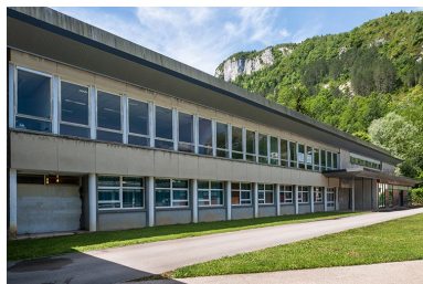
Atelier : façade est. Phot. Jérôme Mongreville IVR43_20143900425NUC4A
