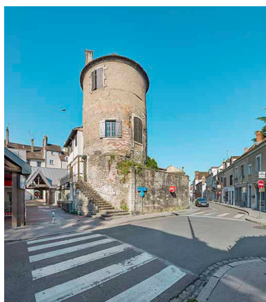
La tour Marcilly. Phot. Thierry Kuntz IVR26_20247100044NUC4A
