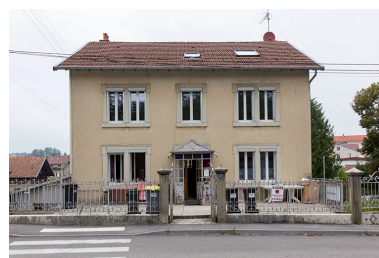
Façade antérieure. Phot. Yves Sancey IVR43_20122502314NUC2A
