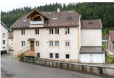
Façade antérieure. Phot. Sonia Dourlot IVR43_20172500413NUC4A
