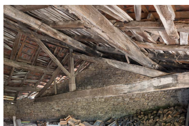
Charpente du cuveau Phot. Pierre-Marie Barbe-Richaud IVR26_20197100257NUC4A
