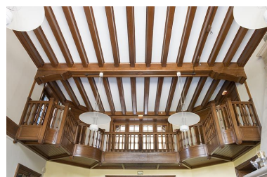
Mezzanine du salon. Phot. Jérôme Mongreville IVR43_20112501512NUC4A
