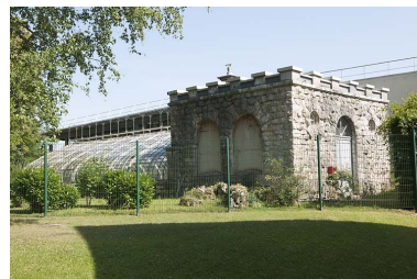
Serre. Phot. Jérôme Mongreville IVR43_20112501514NUC4A
